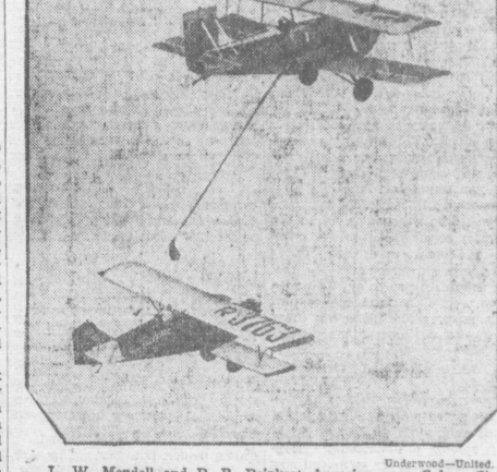
L. W. Mendell and R. B. Reinhart, hovering over Culver City, Calif., in their biplane "Angeleno" have broken all records for refueling endurance flights. Picture gives a striking view of actual contact being made between "Angeleno" and its refueling plane.
