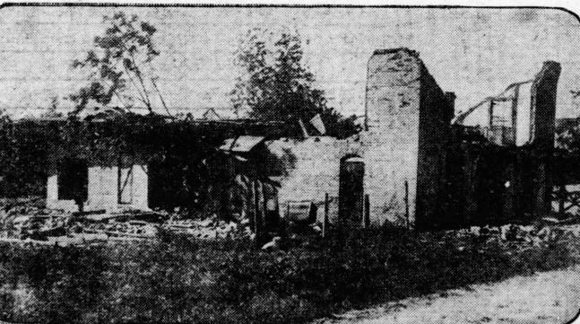
The ruins of a brick building near Cochran, Ga., which was destroyed by a terrific twister that took scores of lives and injured hundreds, doing untold property damage.
