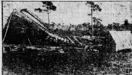
A typical scene of hurricane damage. This view, taken at Greenacres, Fla., after the disastrous storm of February, 1926, shows how homes collapse under the fearful impact of madly speeding currents. Greenacres is 10 miles southwest of Palm Beach, one of the Florida cities hardest hit by the recent hurricane.
