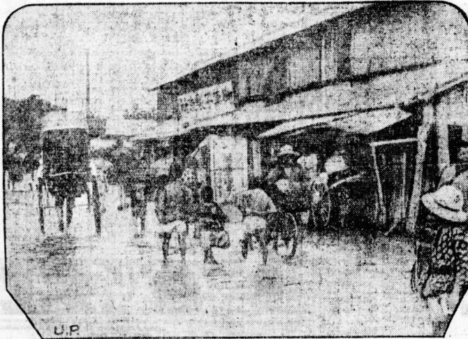
Enormous property damage was done by floods following severe rainfall in Saitama Prefecture, Japan. Here is a scene in Kumagaya, almost completely inundated by the storm waters. Kawaguchi also was hard hit.
