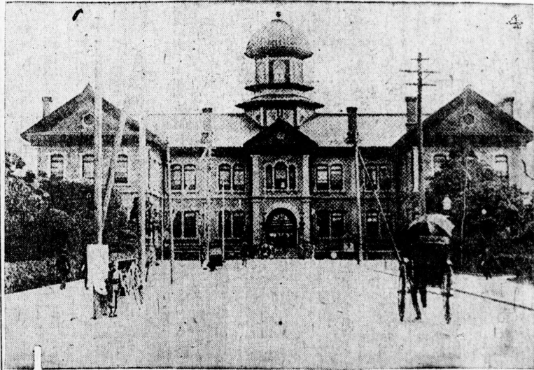
關稅濱橫るたし失燒壞倒 (Caption for the photograph)
